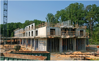
George Mason University: Construction Site
