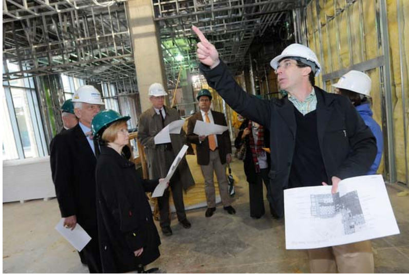
Mason President and Mrs. Allen Merten, left, recently toured the construction site. Andrew Klamon, vice president of development for Concord Eastridge, the project's development company, pointed out some of the facility's features. Creative Services photo
